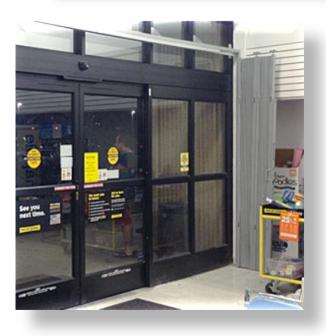
In a storefront location with long and large banks of windows that must be secured with window gates, instead of attaching each gate to the window mullions, the Top Track System lets you secure the gates to each other, not the window frames. As a result, each leading edge of the window gate has a heavy duty roller bearing that feeds into the aluminum top track secured above the window.
